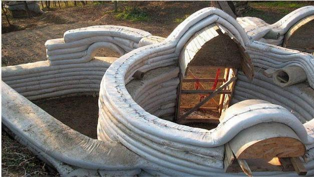
We lay strands of galvanized **barbed wire** between the superadobe rows, which keep the layers together (like mortar) and increase the tensile strength of the structure.
